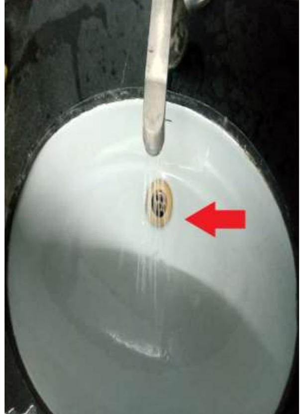
Used reducer to tap water for purpose of washing of utensils, hands etc which reduces flow of water and ultimately saves the water.
